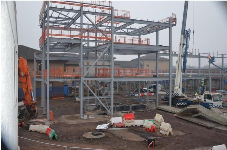
**Image 1: Steelwork to 2-storey element and lift pit (end of Atrium) with steelwork to single-storey element beyond (Children's Inpatients, Oncology, and Outpatients)**
