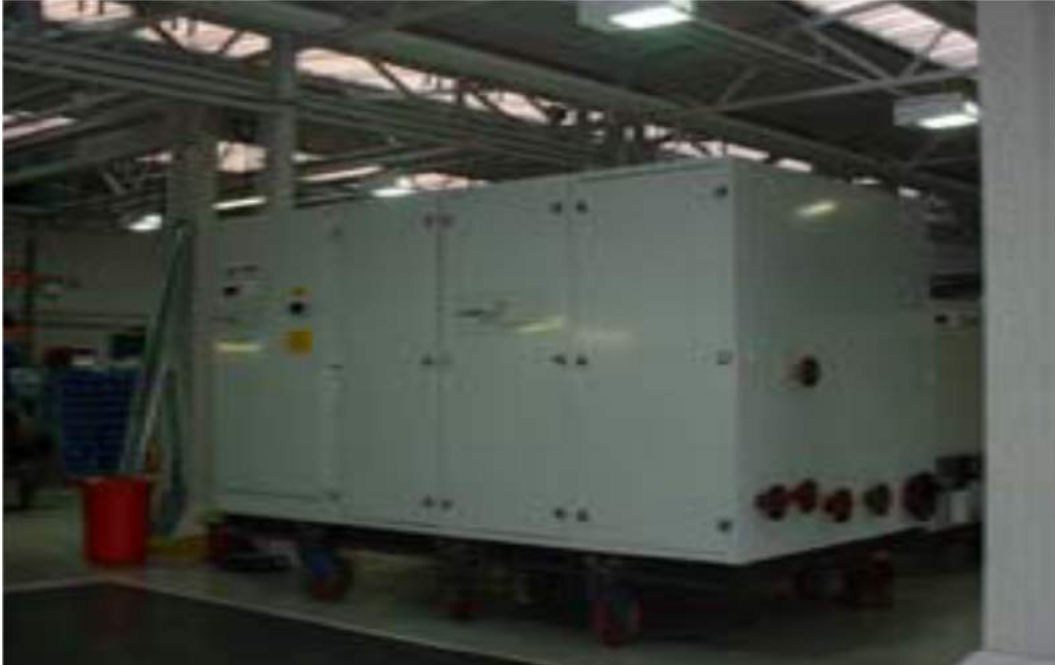
Figure 17- Containerised CHP Plant
