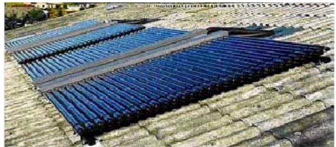
Figure 10 - Evacuated Tube Solar Water Heating
