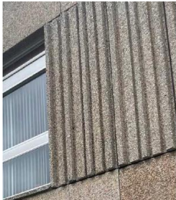
Original Building Materials
