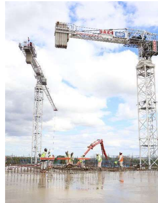
Final concrete pour of area 1 taking place
