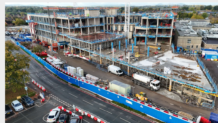
Final concrete frame to complete
