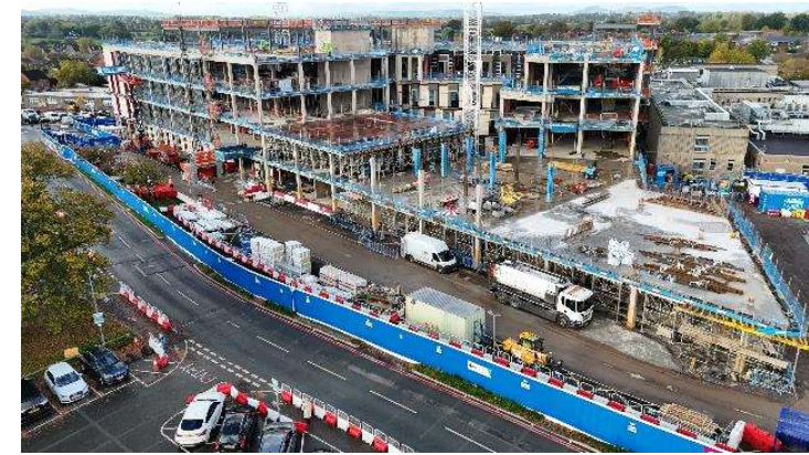
Final concrete frame to complete
