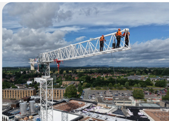
First tower crane being dismantled
